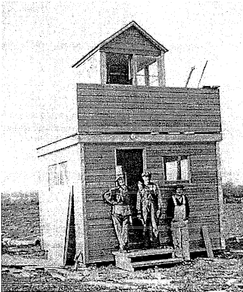
Figure 1 - Builders Fred Lambert, Adolph German, Don Woodward, in front of nearly completed Civilian Aircraft Observation Post, October 1942
