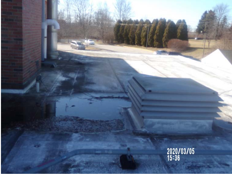
Roof A-North side, looking West
