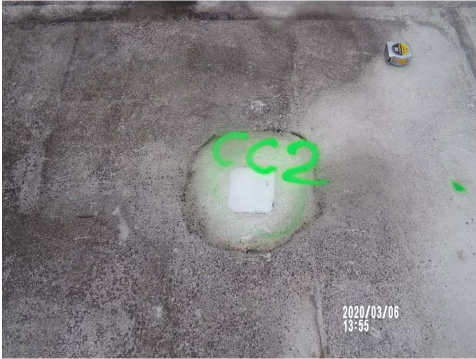
Roof A-Core cut #CC2 repaired, looking East
