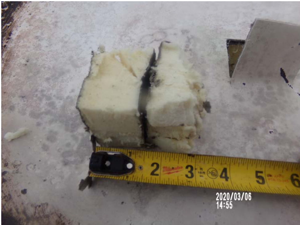
Roof B-Core cut #CCB1 (Dry)
