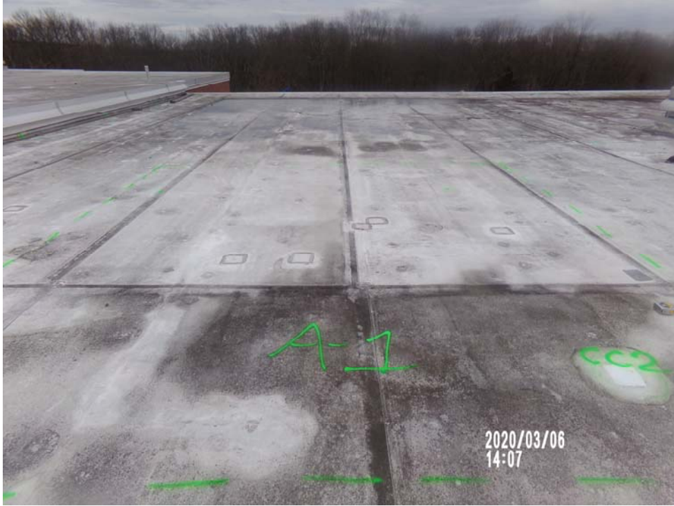
Roof A-Wet area A-1, looking East
