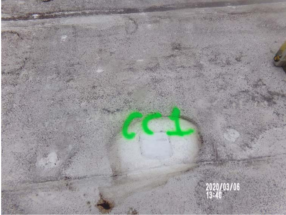
Roof A-Core cut #CC1 repaired, looking East
