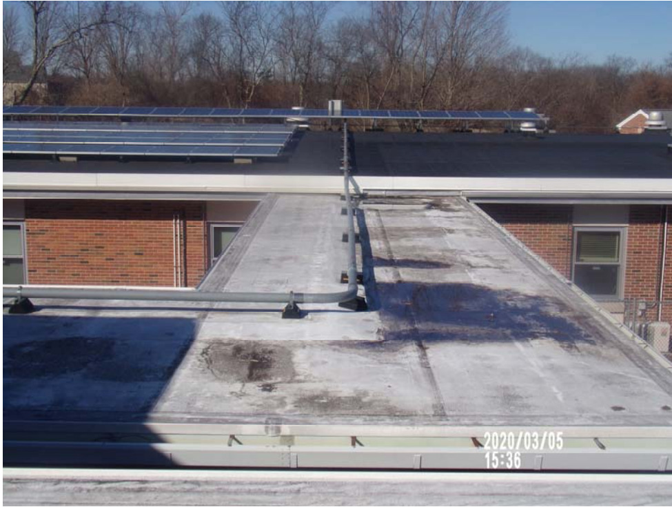
Roof B-Looking North
