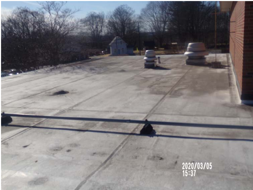
Roof A-South side, looking West
