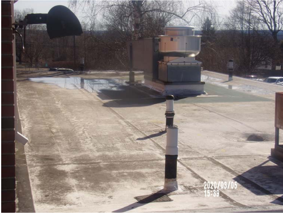
Roof E-Looking South
