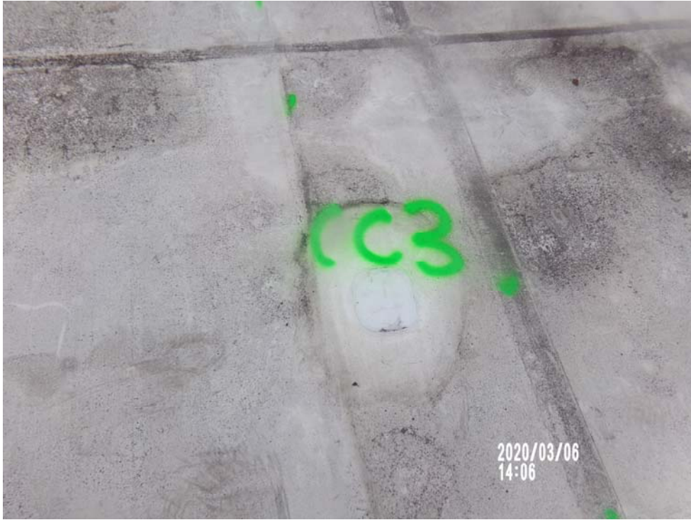
Roof A-Core cut #CC3 repaired, looking East
