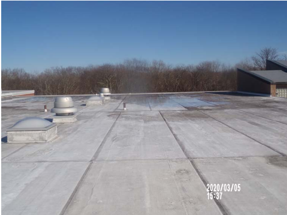
Roof A-Center, looking East
