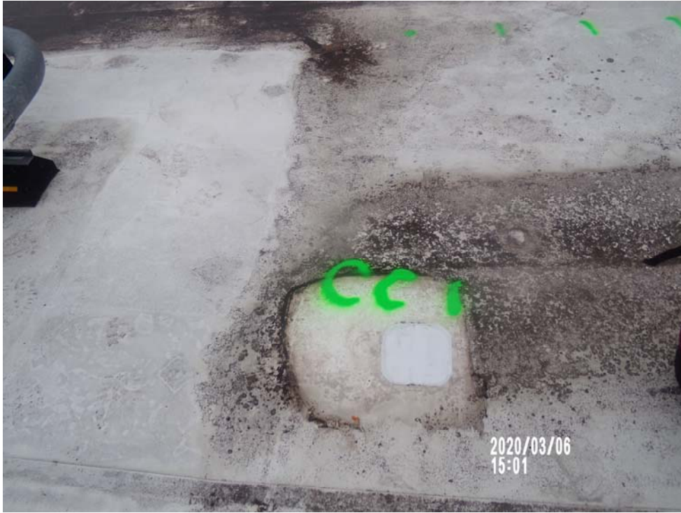
Roof B-Core cut #CCB1 repaired, looking East
