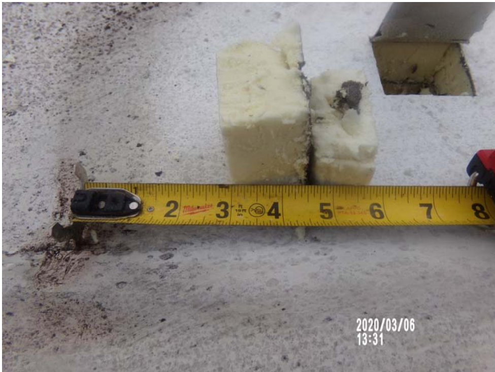
Roof A-Core cut #CC1 (Dry)
