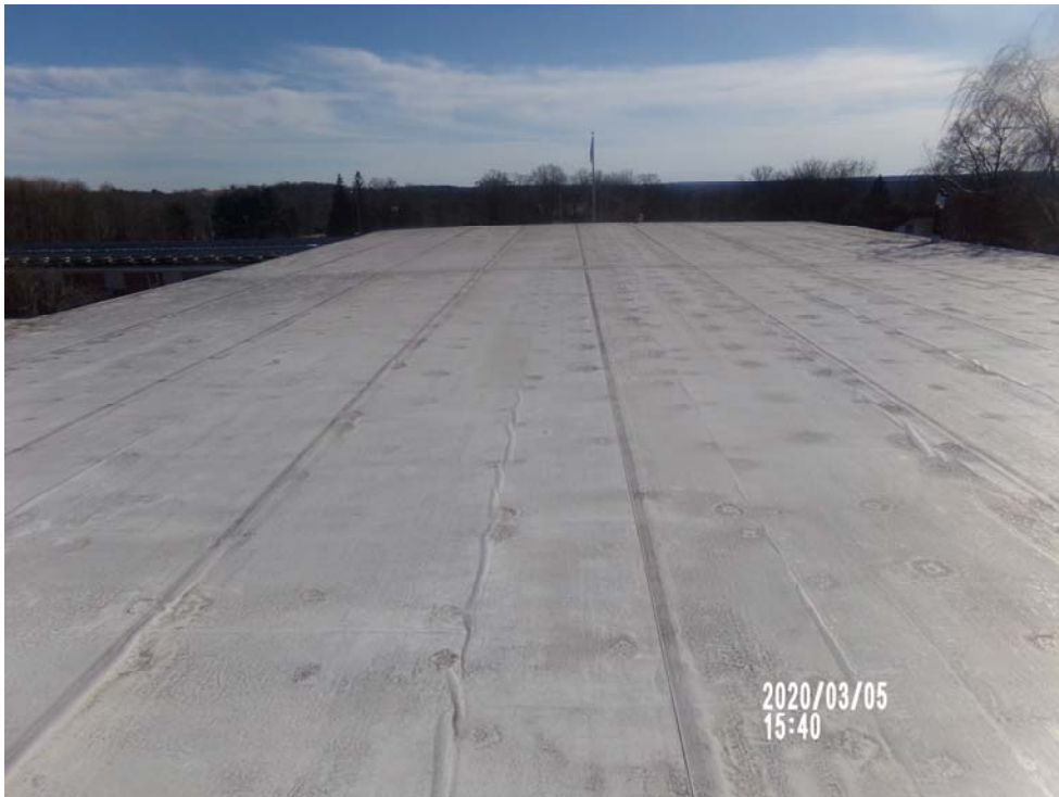
Roof D-Looking South
