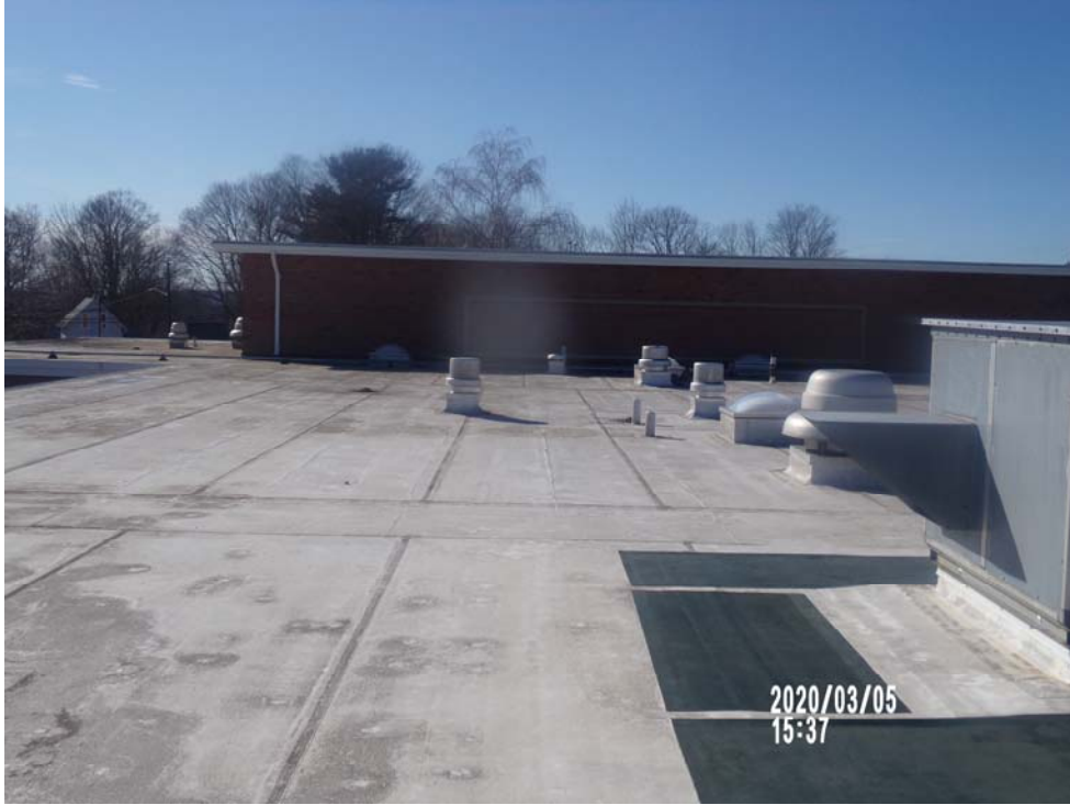
Roof A-Center, looking West
