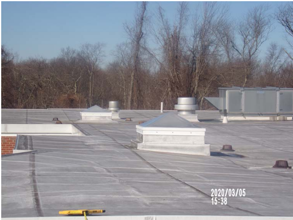
Roof C-Looking North
