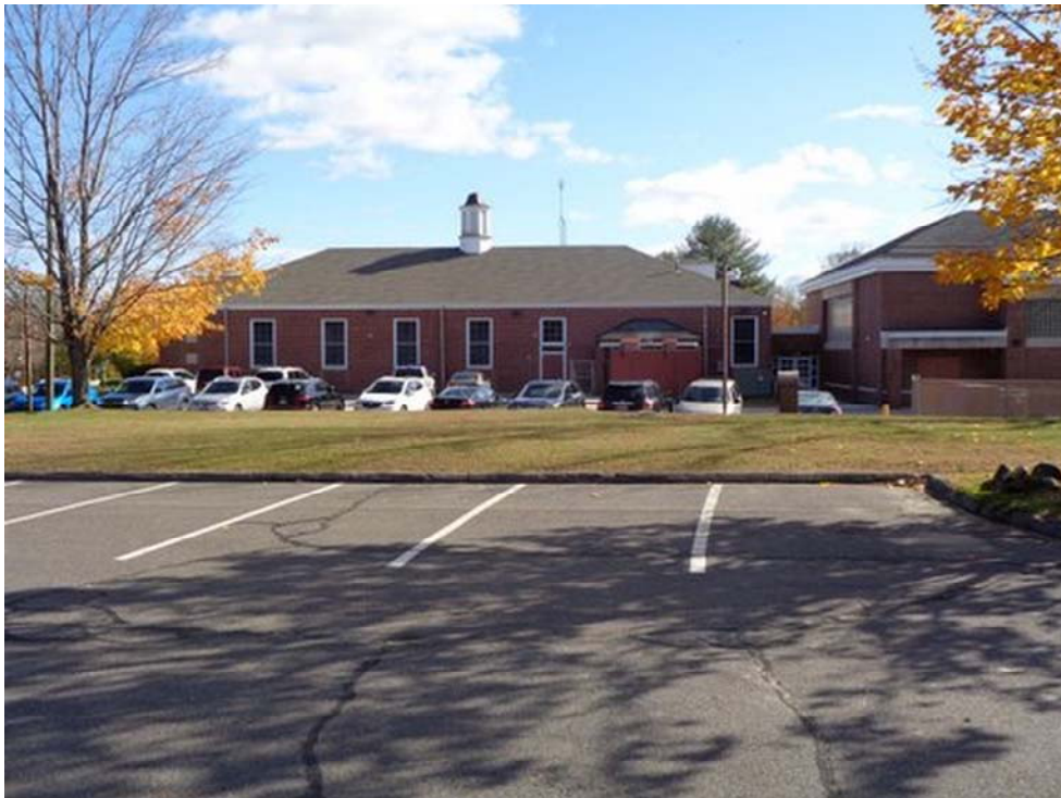
North side of building, looking South
