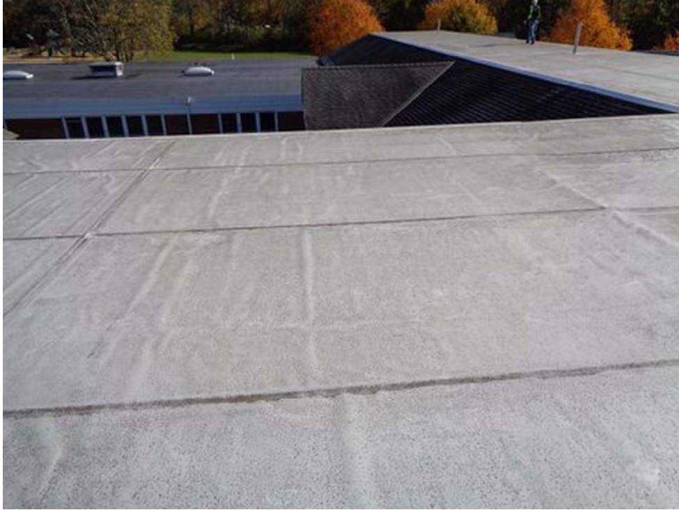
Roof A-Overview, looking South
