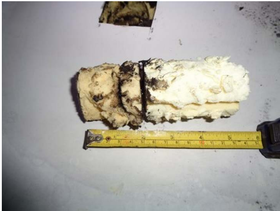
Core Cut #CC1-TPO, 1 1/2" Polyisocyanurate, 1/2" Polyisocyanurate, 3" Polyisocyanurate and a metal deck. (Wet)
