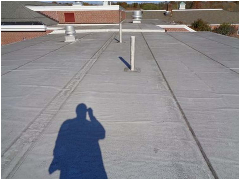
Roof A-Overview, looking East
