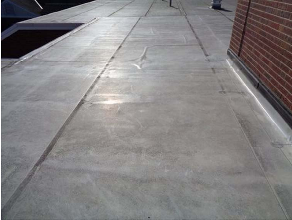
Roof D-Overview, looking West
