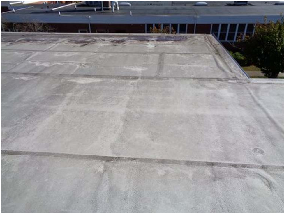
Roof D-Overview, looking South
