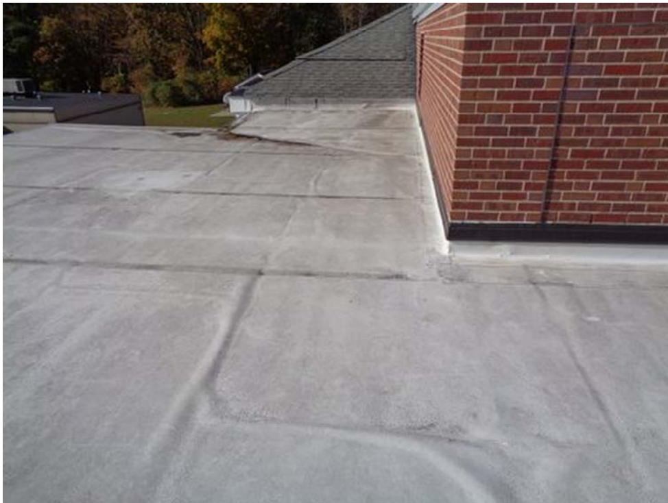
Roof D-Overview, looking North
