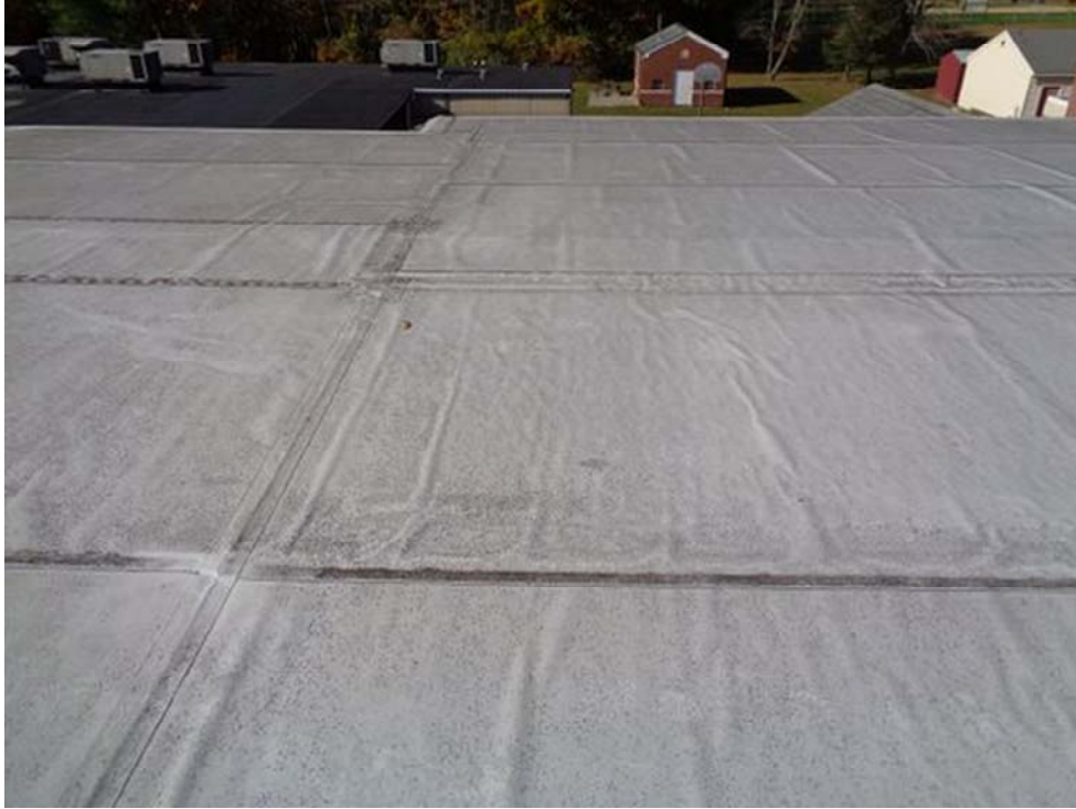
Roof A-Overview, looking North
