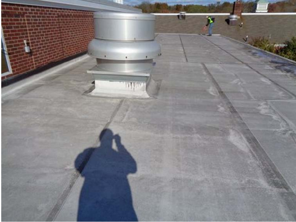
Roof D-Overview, looking East
