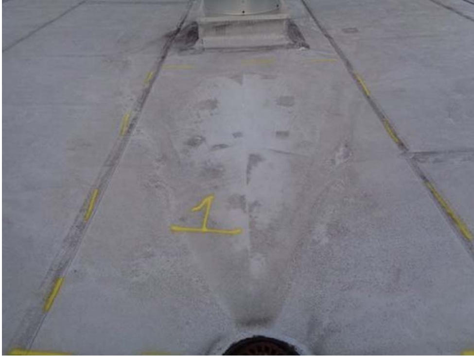
Roof B-Wet area #1, looking East
