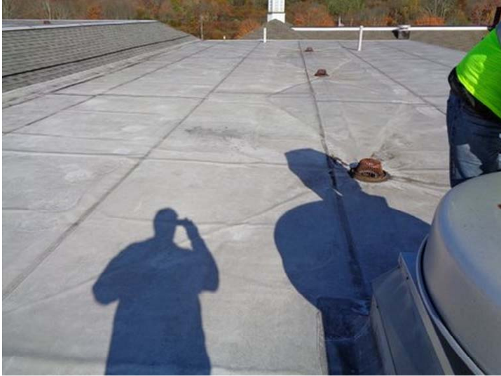
Roof E-Overview, looking East
