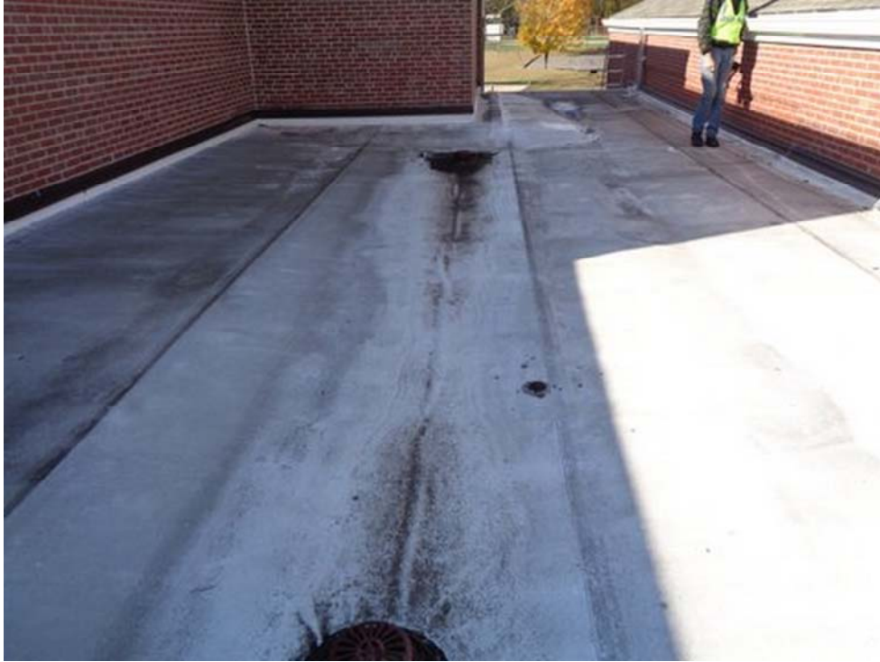
Roof C-Overview, looking North
