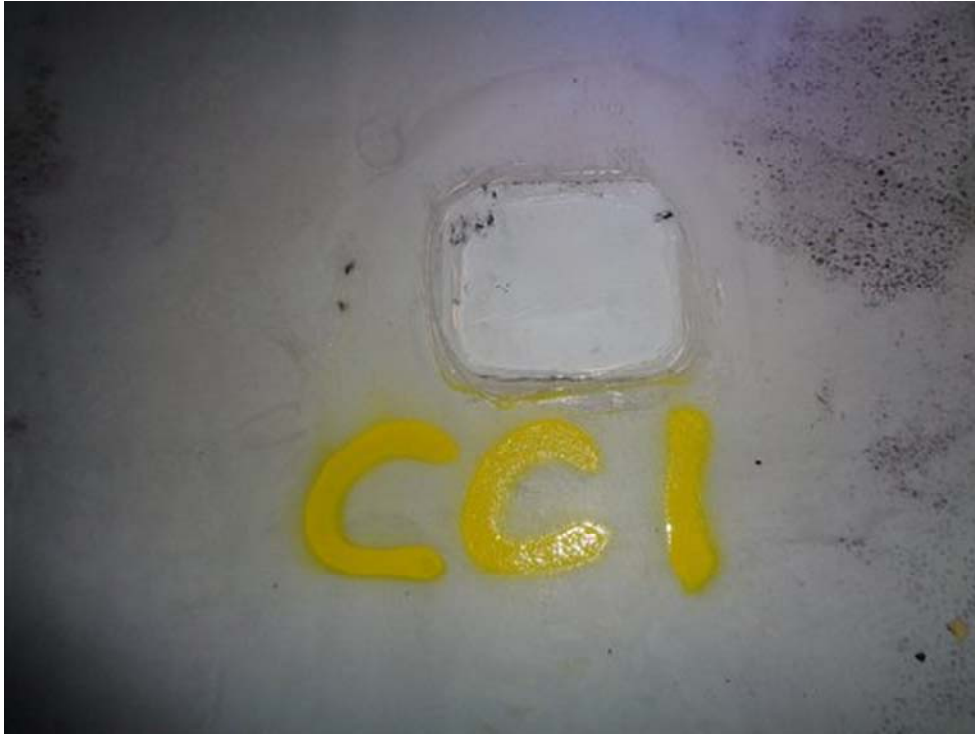
Core Cut #CC1 repaired
