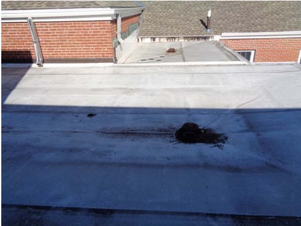
Roof C-Overview, looking East
