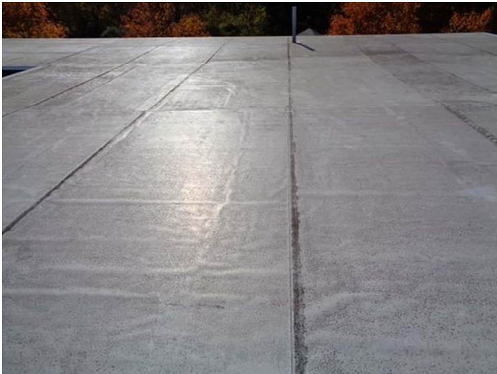
Roof A-Overview, looking West
