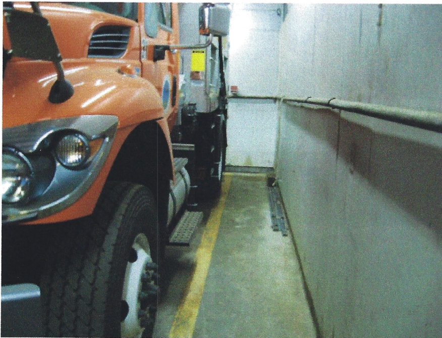
Figure 17: Minimal aisle clearances endanger equipment and building.
