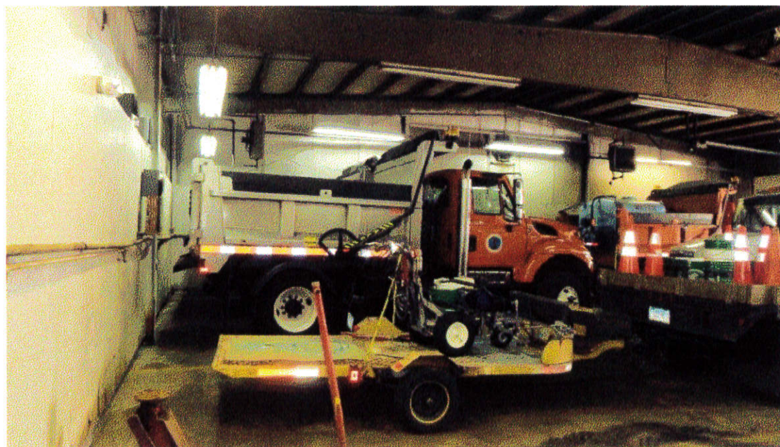
Figure 21: New vehicle storage bays should be higher than the existing bays to facilitate access to equipment without damaging building structure.
