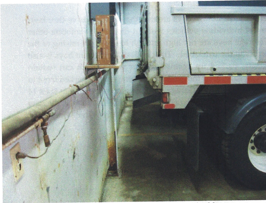
Figure 18: Limited clearances endanger wall surfaces, building structure and wall mounted utilities as well as limiting passage of personnel.
