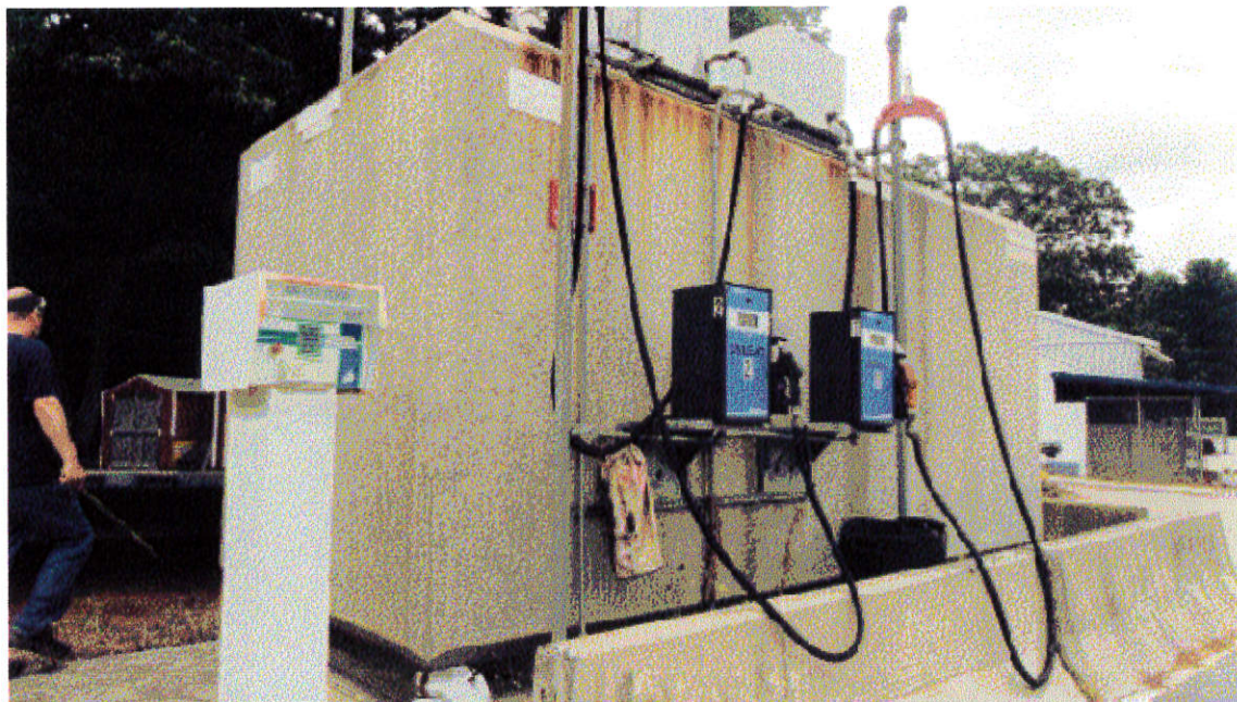
Figure 6: The existing fueling island can be renovated with new dispensers, pumps and fuel management system.
