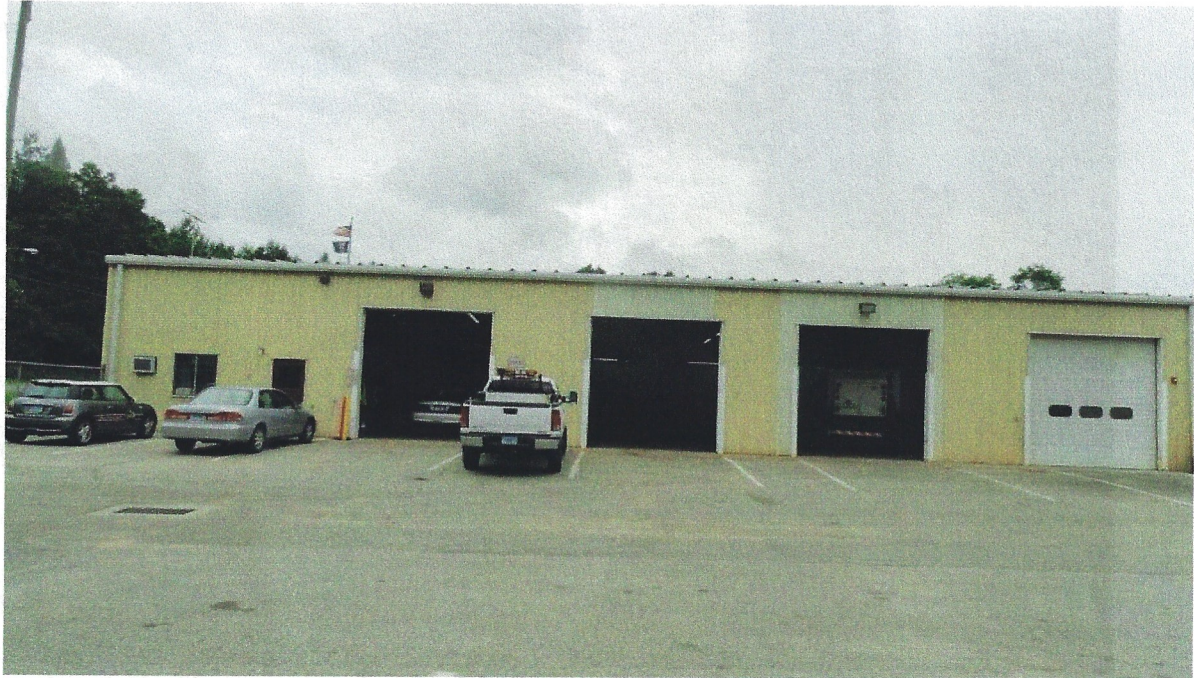
Figure 11: The main building at 550 Old Colchester Road is a metal building housing equipment bays, maintenance bays, administration offices and support facilities.
