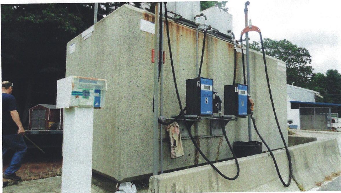
Figure 6: The existing fueling island is in good repair with new tanks and dispensers.
