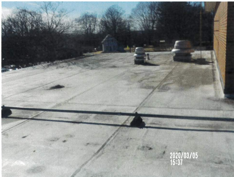
Roof A-South side, looking West
