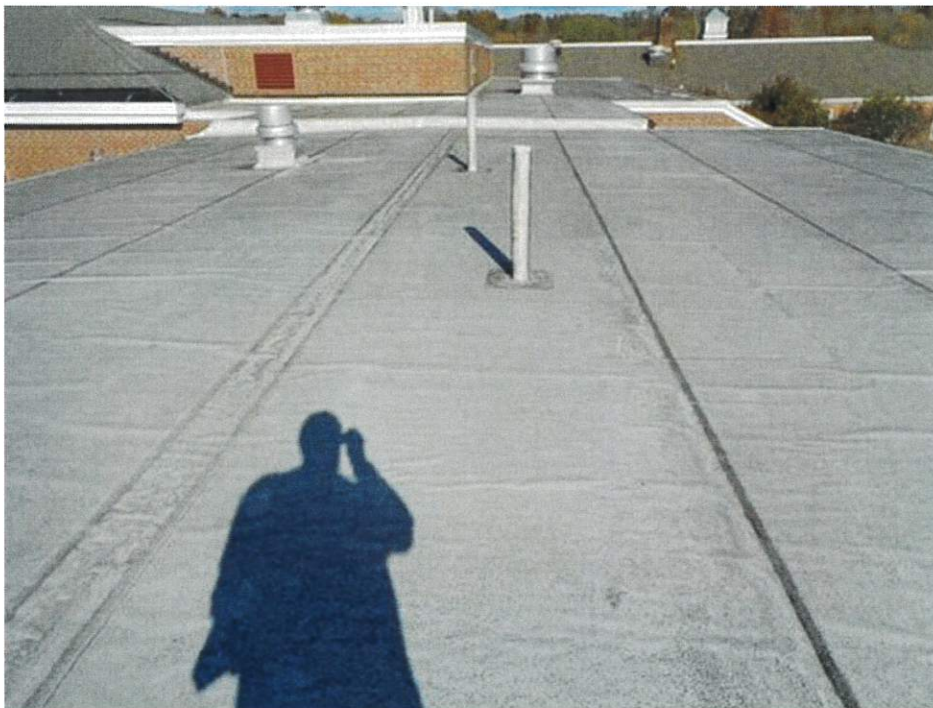
Roof A-Overview, looking East
