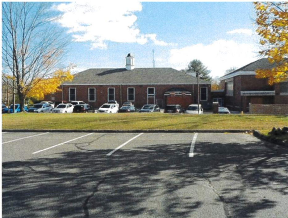
North side of building, looking South
