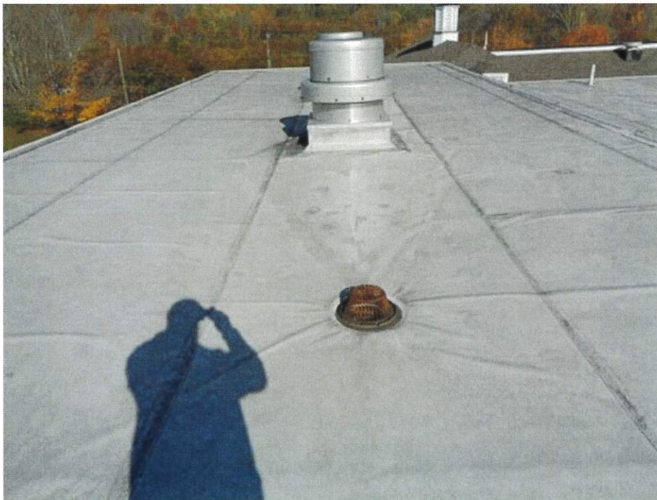
Roof B-Overview, looking East
