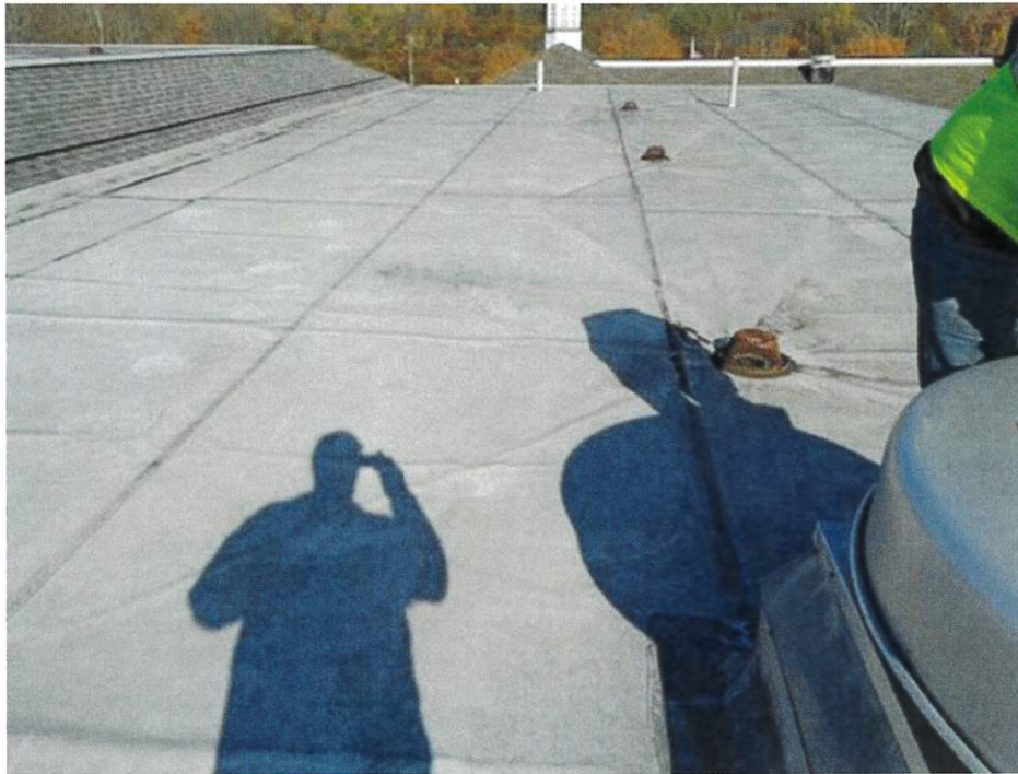
Roof E-Overview, looking East
