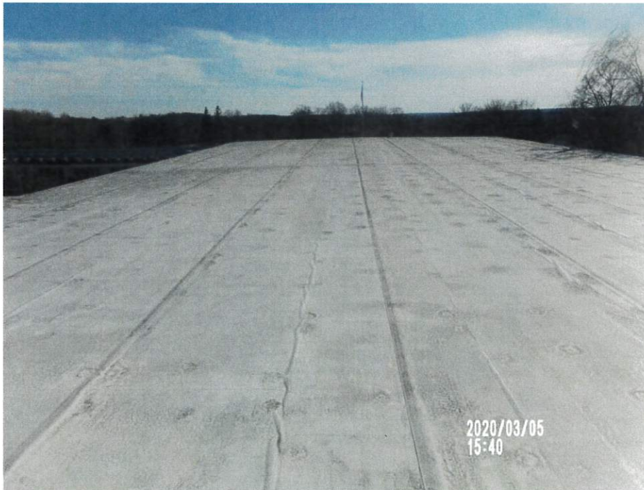
Roof D-Looking South
