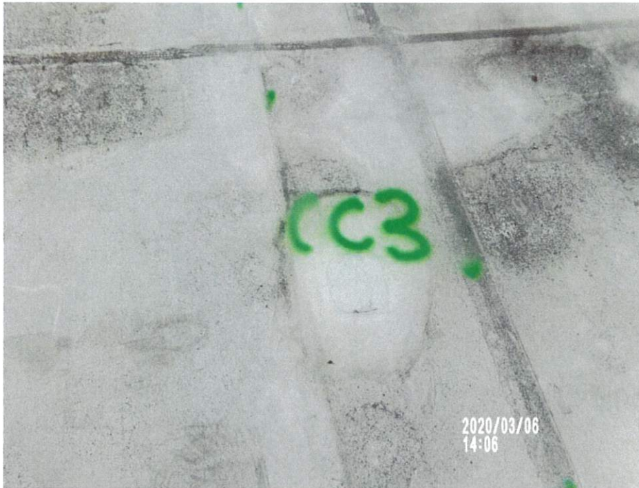
Roof A-Core cut #CC3 repaired, looking East
