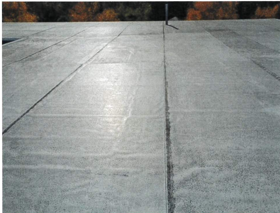
Roof A-Overview, looking West
