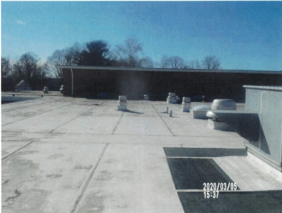
Roof A-Center, looking West
