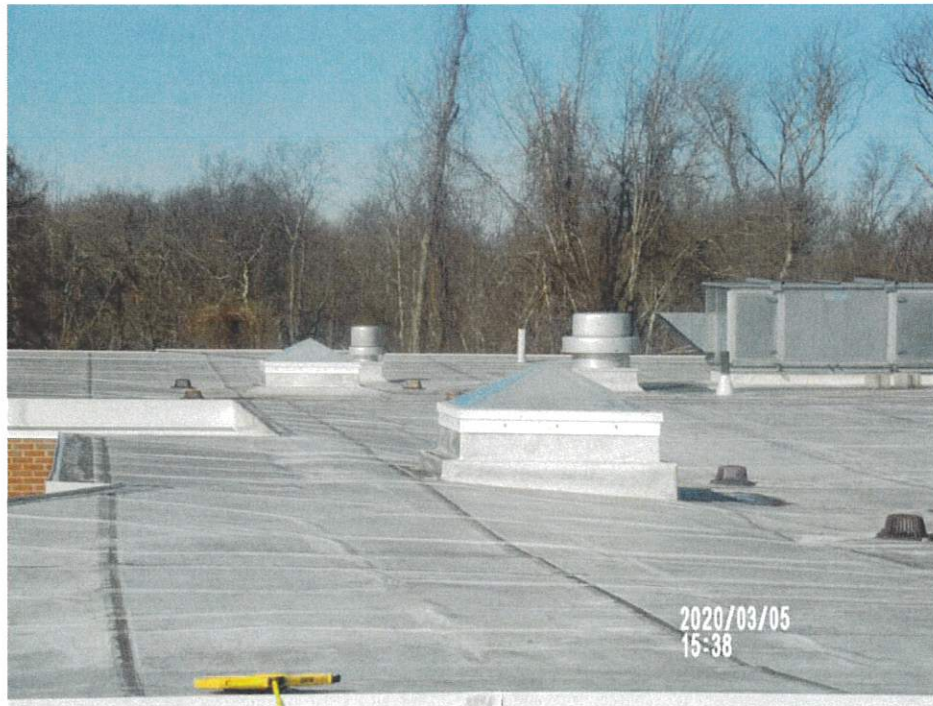
Roof C-Looking North
