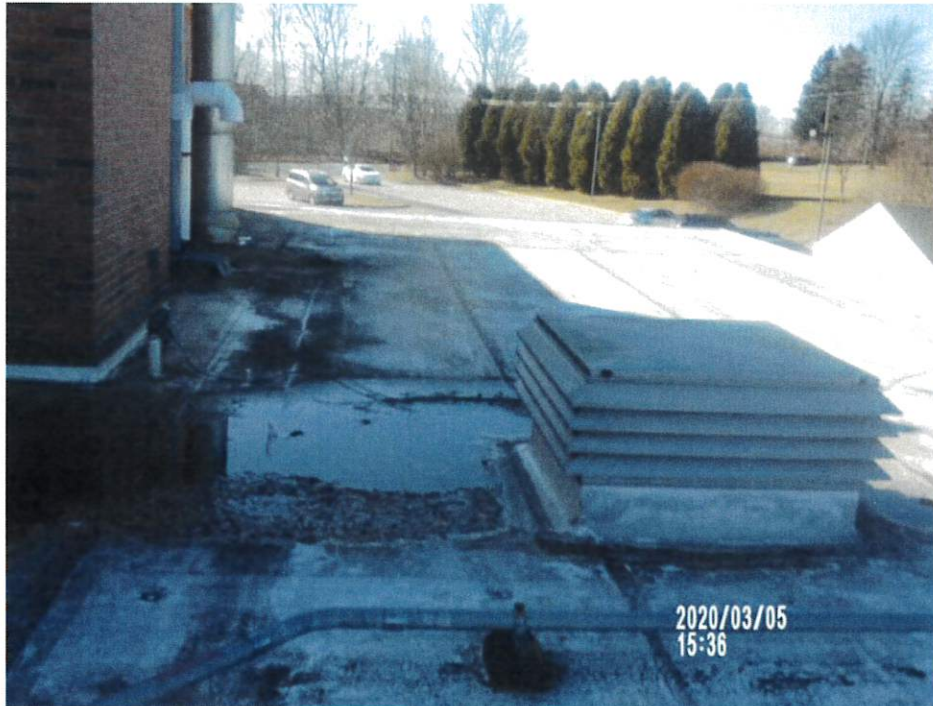
Roof A-North side, looking West
