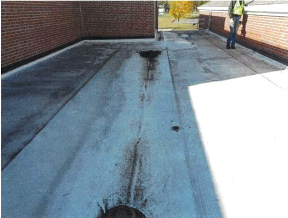
Roof C-Overview, looking North
