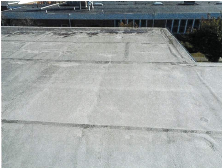
Roof D-Overview, looking South
