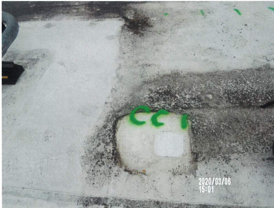
Roof B-Core cut #CCB1 repaired, looking East
