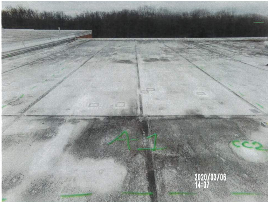
Roof A-Wet area A-1, looking East
