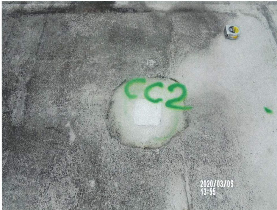
Roof A-Core cut #CC2 repaired, looking East
