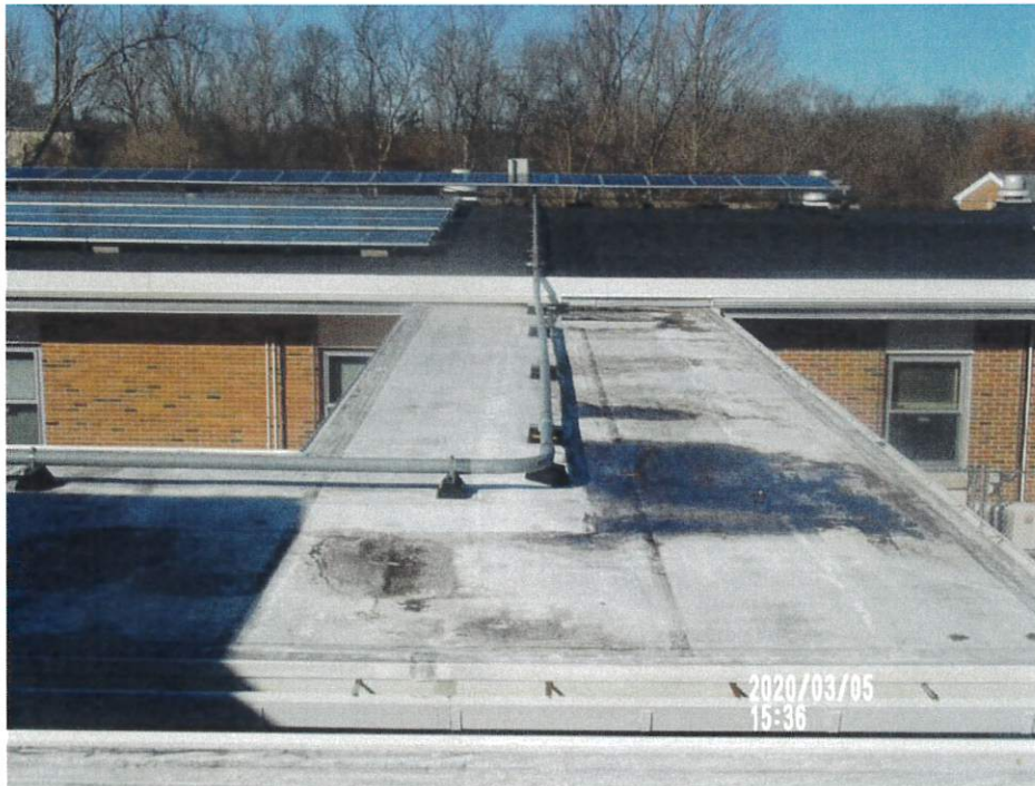
Roof B-Looking North
