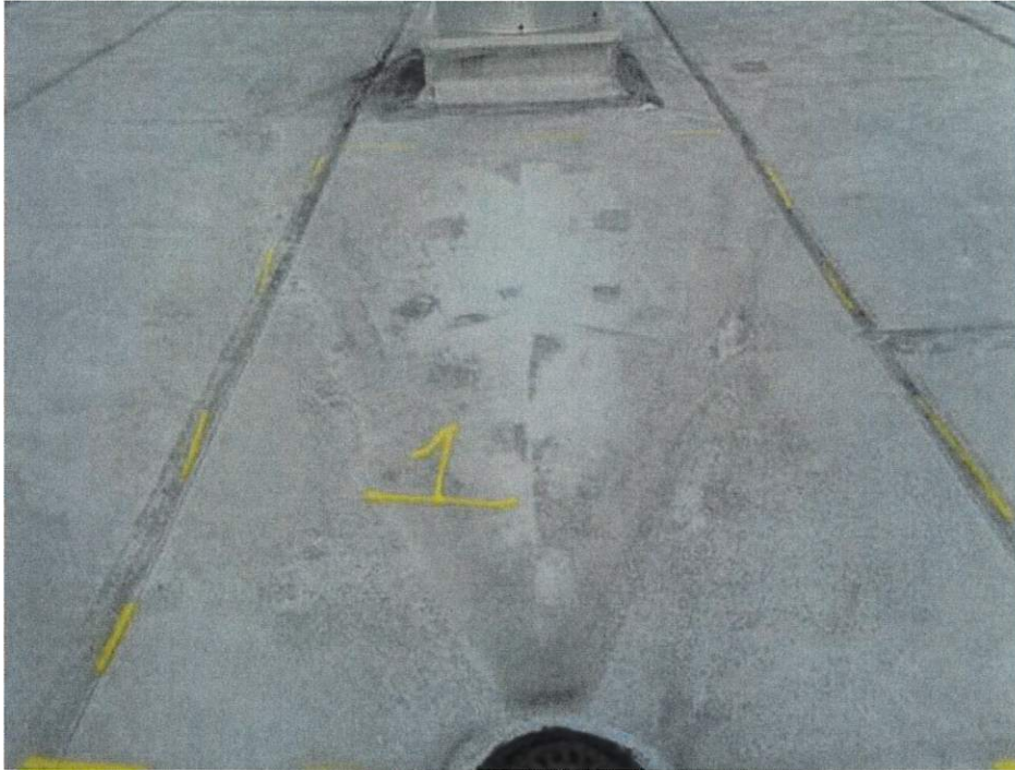
Roof B-Wet area #1, looking East
