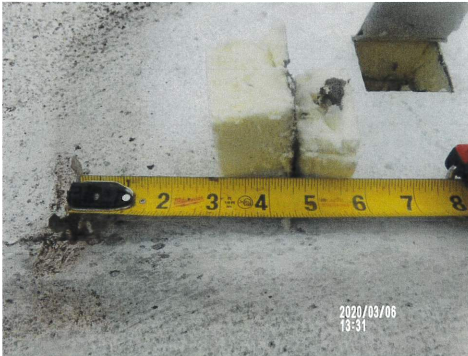
Roof A-Core cut #CC1 (Dry)
