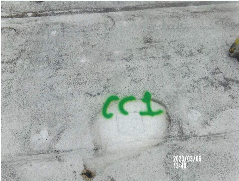
Roof A-Core cut #CC1 repaired, looking East
