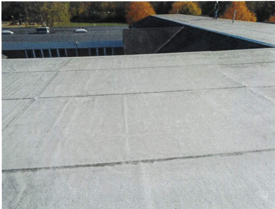
Roof A-Overview, looking South
