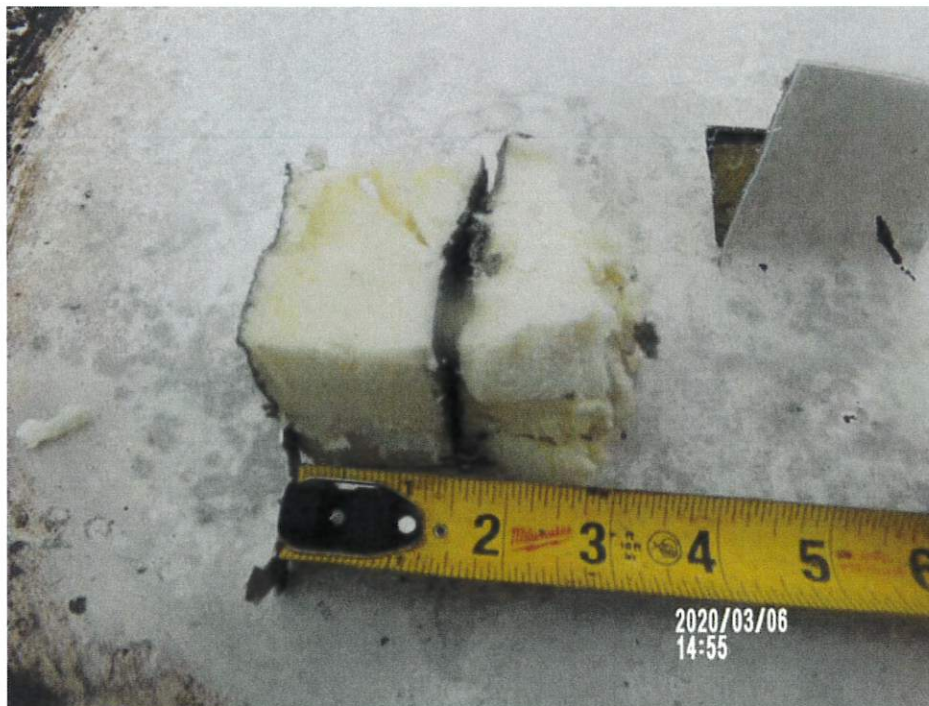
Roof B-Core cut #CCB1 (Dry)
