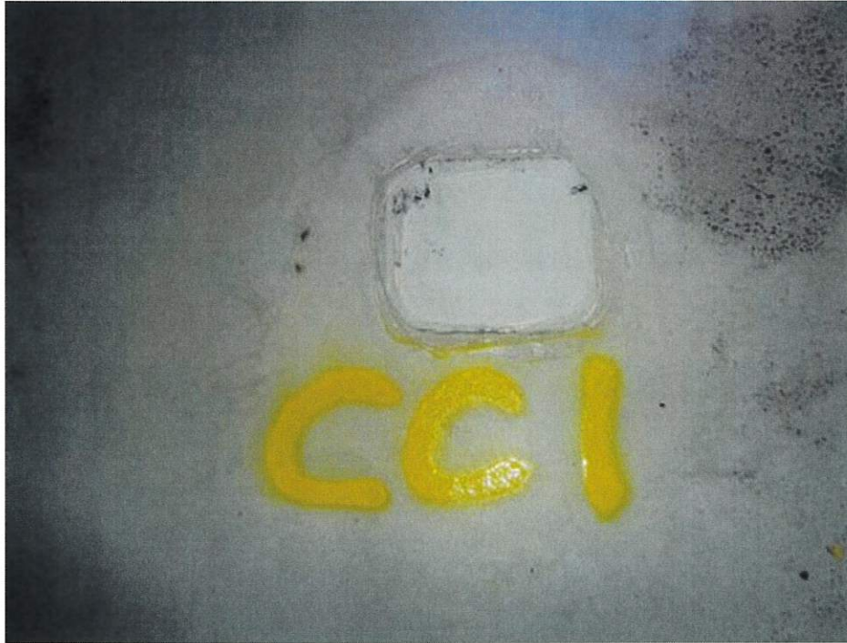
Core Cut #CC1 repaired
