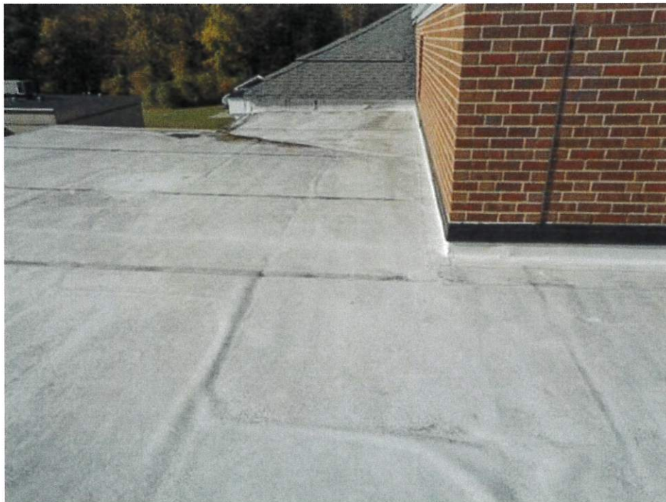
Roof D-Overview, looking North
