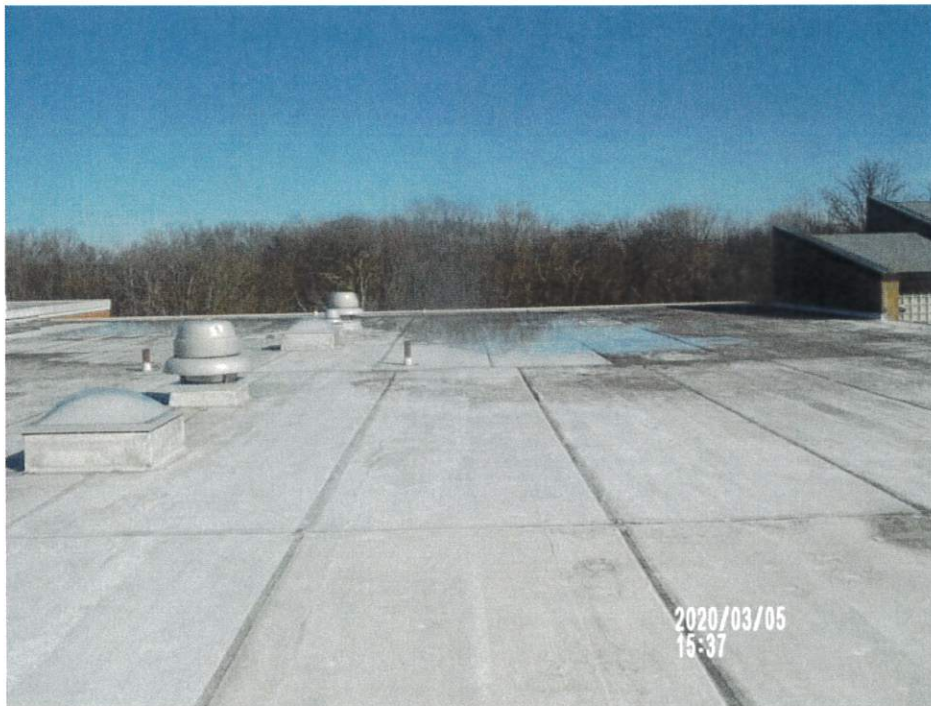
Roof A-Center, looking East
