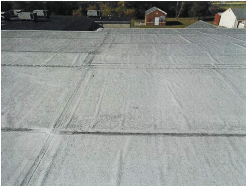
Roof A-Overview, looking North
