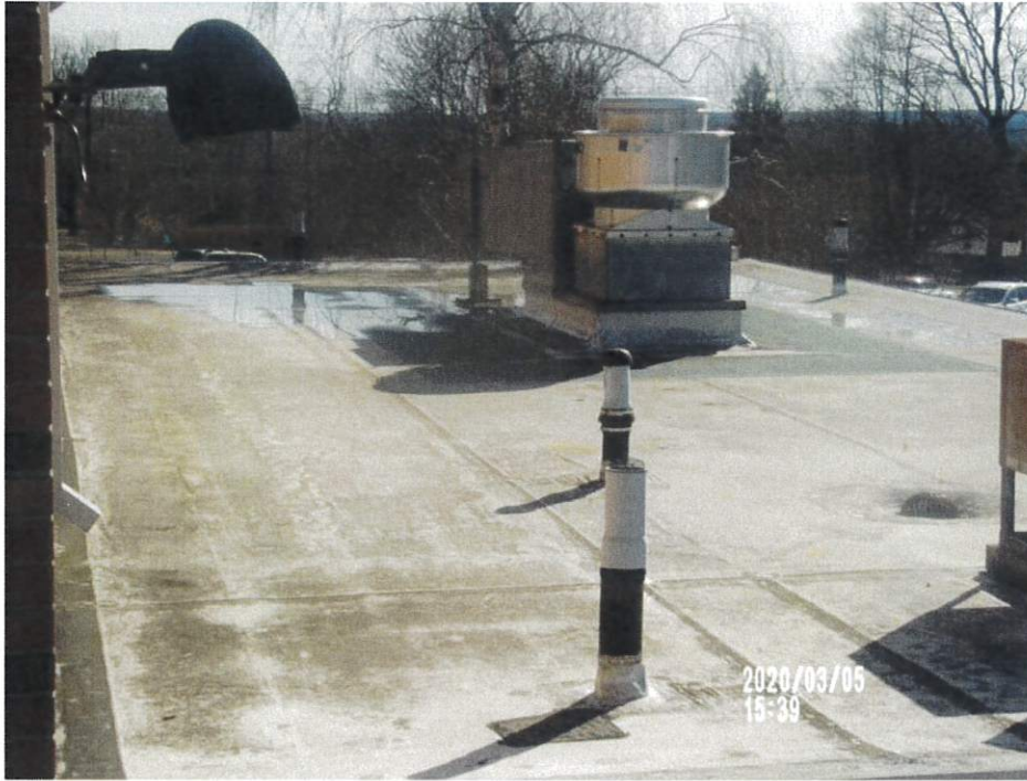
Roof E-Looking South
