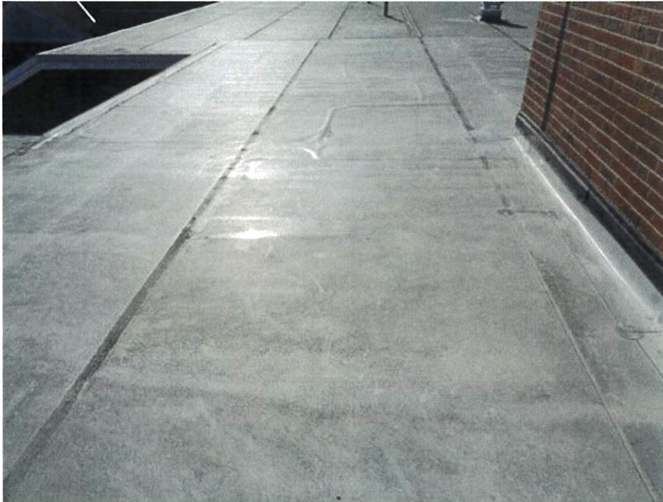
Roof D-Overview, looking West
