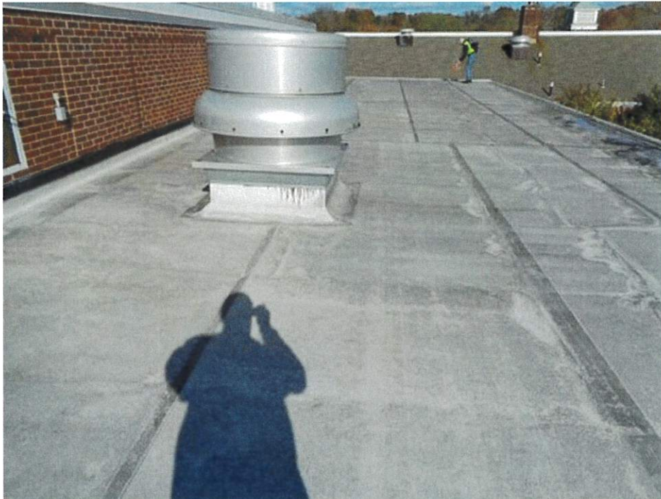
Roof D-Overview, looking East
