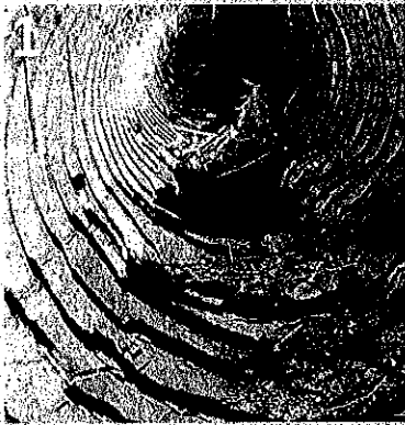
1 Blocked storm pipe
