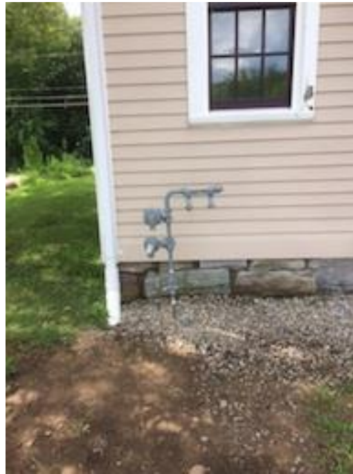
Natural Gas Brought to Peters House
