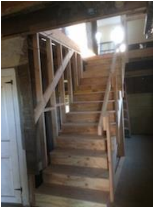
Work Staircase to 2 nd floor.
