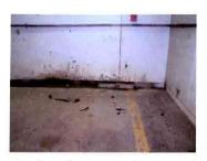
The south side wall of the garage bays have been damaged by vehicle impacts. Both the metal wall panels and the concrete masonry units should be replaced. Due to the close proximity of the metal siding to the ground, the siding has rusted. This is evident especially around the doors. Many areas along the bottom edge of the wall panels are rusting. Replacement of the wall panels and insulation is recommended. There are products that have
