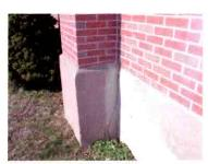
It has been observed when it is raining, water from the roof overflows the gutter and is creating a trough on the ground along the building. This is caused by debris in the gutters and downspouts being clogged. The debris is mainly caused by leaves from the trees to the West. To prevent further ground erosion, maintenance costs and to extend the life of the roof, gutter guards should be installed. This will allow debris to fall off of the roof and reduce the maintenance cost associated with
