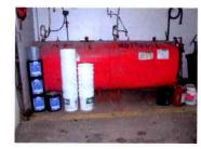
The motor oil tanks located in the garage area should be protected from vehicle impact by the installation of bollards. The potential exists for a vehicle to come in contact with one of the tanks and either knock it over or rupture the side, spilling oil all over the floor. However, the installation of bollards will further restrict the use of the bay.
