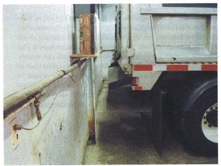
Figure 18: Limited clearances endanger wall surfaces, building structure and wall mounted utilities as well as limiting passage of personnel.
