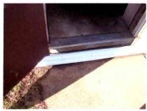
mechanical room has an exterior door and the oil lines run under the door. This is a tripping hazard and is also subject to damaging the piping system. The piping is required to be protected from physical damage.
