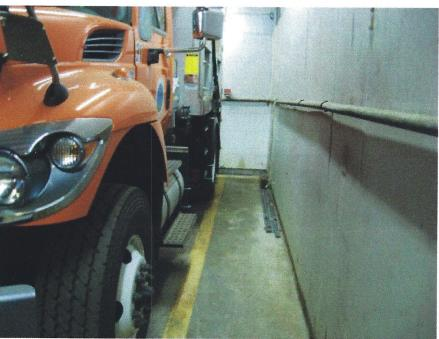
Figure 17: Minimal aisle clearances endanger equipment and building.
