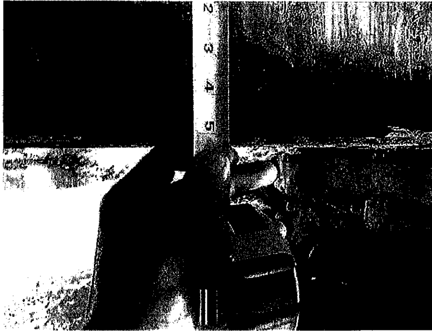
Beam # 3 south face bottom flange with section loss.
