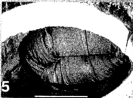
5 Liner inverting out the end of the pipe
