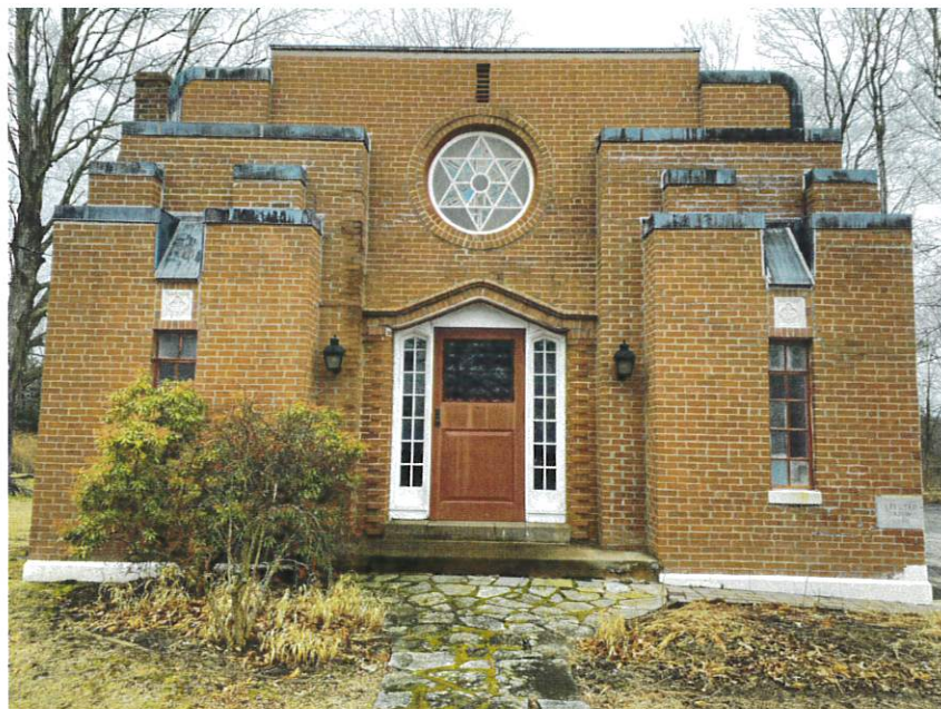
Synagogue, front view, Izzy Turshen, Architect, Hebron resident
